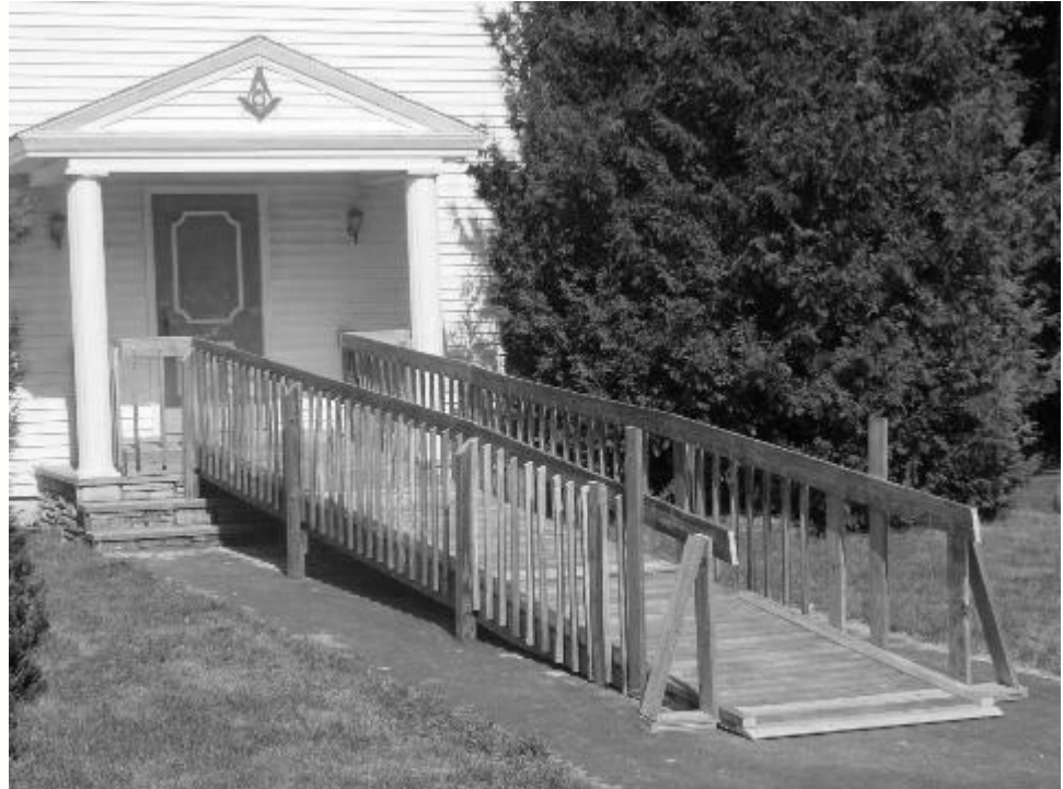
Tyrian Lodge now has a new handicap ramp
